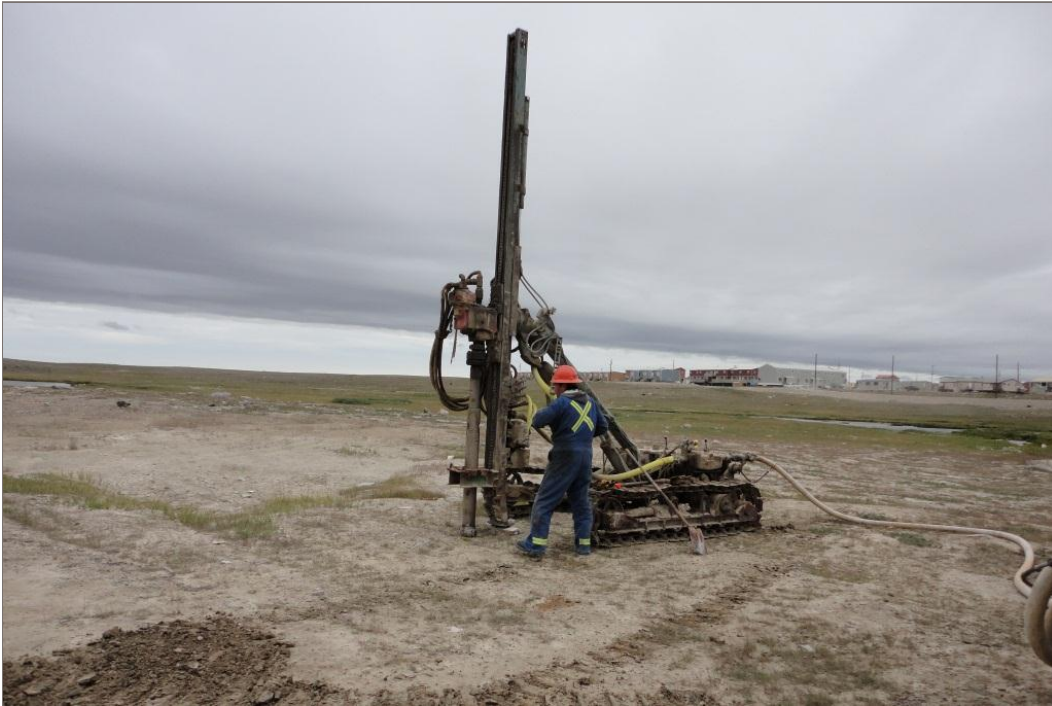
Photo 3: Air-rotary drill at Site A Probehole 01, looking north.
